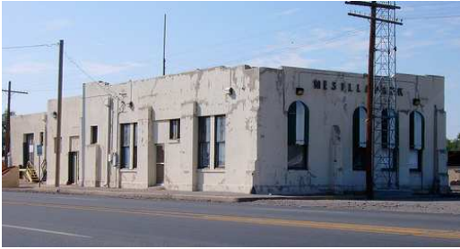
Old depot at Mesilla Park Source: http://flickr.com/photos/99491151@N00/2894197926/
