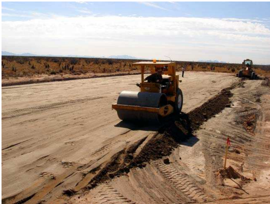
Spaceport site – grading activities http://www.space.com/images/060323_spaceport_bdoze_02.jpg
